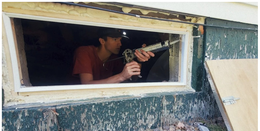
▲ Weatherization crew insulating a Vermont home.
